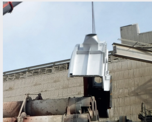
Clinker cooler hood being lifted into place
