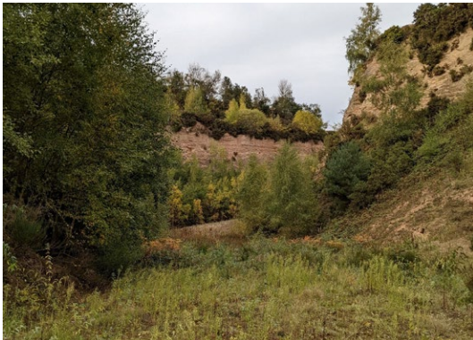
Ongoing restoration work at Bestwood II Quarry
