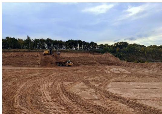
Quarry equipment extracting the sandstone at the face
