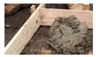
**4. Completing the Foundation** – Once the foundation has cured for the time recommended on the bag, remove the shuttering.
