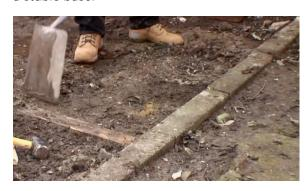
**3. Mix and Pour your Concrete** - Mix ready-to-use Blue Circle High Strength 40N (or Multi-Purpose Concrete) as directed on the bag and pour into the shuttering, ensuring the surface is level.
