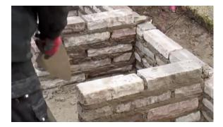
Insert metal pegs into the mortar to support the cooking surface at the appropriate height.
