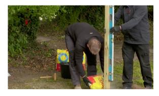
5. Fixing the panels - Once the first post has set, recheck the measurements and position for the next post hole using a fence panel. Repeat the installation process above for fixing the next and subsequent posts. Clean your tools promptly after finishing to prevent any material from hardening on them.
