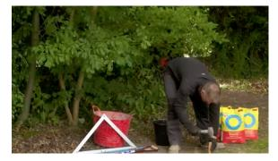
**3.** Check the Position - Insert the post in the hole to double check the hole depth and width to make sure both are correct. Remove the post.
