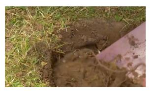
2. Dig the first Hole - Dig the hole for the first post to at least one third of the height of the post being used and about 3 to 4 times as wide.
