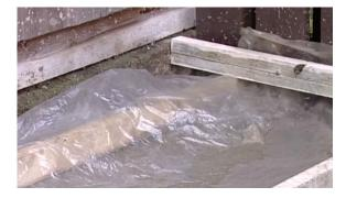
8. **Remove Formwork** - Once the steps have cured, carefully remove the formwork.
