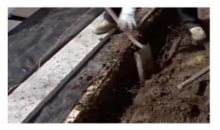
**3.** Add a Gravel Base - To improve drainage and stability pour a layer of gravel into the foundation area. Level and compact the gravel using the tamper.
