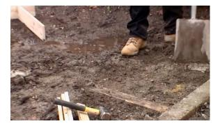
2. Prepare the Area - Prepare the area for the step. If building the step on soil, dig out the required area and use the tamper to compact the soil to ensure a stable foundation.
