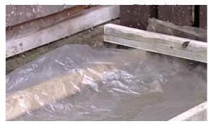
Curing - Cover the concrete with sheeting and allow to cure for at least 7 days before use.
