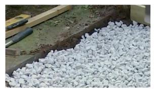
4. Install Formwork - Set up the formwork for the steps using wooden boards. Ensure the formwork is securely in place and follows the planned dimensions for the steps.
