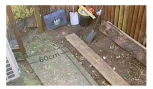
2. Prepare the Area - Dig out the marked path area to a depth of about 6 inches to allow for a hardcore foundation layer and the concrete path upper layer.
