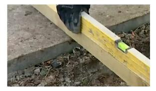
4. Create a solid foundation - Pour a layer of hardcore or gravel into the excavated area. Level and compact the gravel foundation layer using the tamper.
