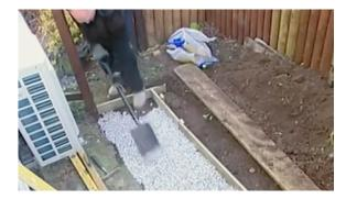
5. Mixing and Laying the Concrete – Following the instructions on the bag, mix the ready-to-use Blue Circle Multi-Purpose Concrete. Place the mixed concrete onto the gravel foundation, spreading it evenly with a shovel and level with a straight edge.
