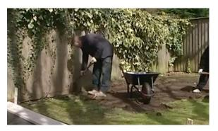
3. Footings for Retaining Wall - Dig a trench to create footings for a retaining wall around the border of the patio. Set levels for the final patio height using wooden pegs and string to ensure it is level and consistent across the area.
