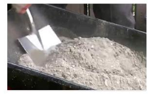
7. Laying Paving Slabs - Mix Blue Circle Mastercrete cement with sand and water as directed on the bag to create the bedding mortar for the slabs. Carefully place the paving slabs using the bedding mortar, starting from one corner and working your way across. Tap each slab into place with a rubber mallet to ensure they are level and secure.
