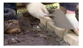
5. Adding a Gravel Base - Pour a layer of hardcore or gravel into the area within the retaining wall. This helps with drainage. Level and compact the gravel.
