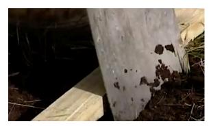
**2.** Level and Compact - Ensure the base is level and compacted. Compact a layer of hardcore for extra stability if required on soft ground.
