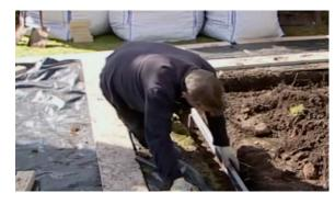
**3.** Laying the Footings for Retaining Wall - Using the instructions on the bag mix the Blue Circle Multi-Purpose Concrete and pour the mixed concrete into the footings trench.
