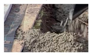
**4. Compacting and Leveling** - Ensure the footings are well compacted. Level the surface with a straight edge. Cover and allow to cure for 7 days.
