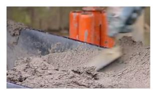
Level and smooth the slab surface with a trowel and straight edge.
