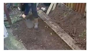
2. Pour out the Slablayer Mix - Pour the dry Blue Circle Slablayer mix from the tub straight onto the prepared ground and rake it level.
