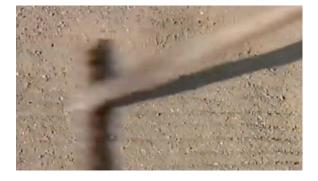
3. Sprinkle with water – Sprinkle the Blue Circle Slablayer with water using the watering can and rake level again.
