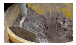
3. Making the repair - Lay the new mortar as required to replace the bricks. Finish the repair using the pointing tool and cover with plastic sheeting for at least 24 hours to allow to cure fully.
