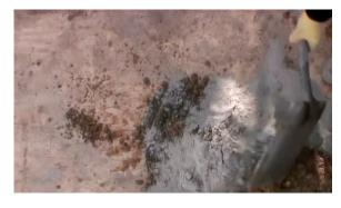
Forming a crater in the centre add some of the water, pulling the dry material inwards onto the water and mix together.
