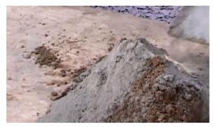
Be sure to add all the water as per the instructions and mix thoroughly until uniform in consistency and colour before laying the concrete
