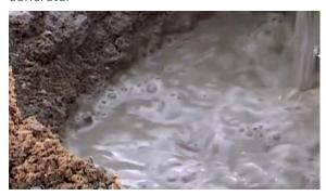
Once fully mixed, use the concrete promptly to ensure optimum workability.
