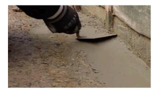
**4. Curing** - The new quick set concrete will cure in about 30 minutes. Re-wet the repair after 2 hours using the watering can.
