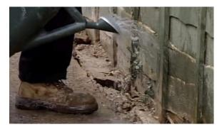
2. Apply the Repair Concrete - Pour the Blue Circle Quick Repair mix into the damaged area. Spread and level the mix then sprinkle water over, allowing it to soak in but not puddle.
