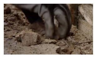
Wet the damaged area with water before applying the concrete repair mix. This helps improve the bond between the existing concrete and the new repair material.
