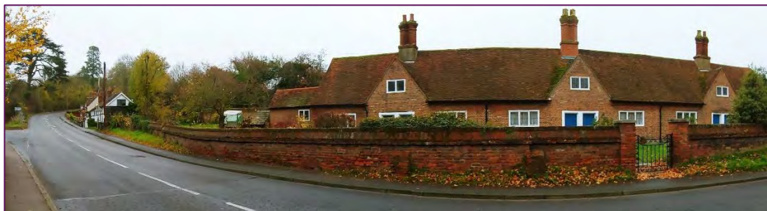
Figure 11: The Baish Almshouses looking south along Roydon Road
