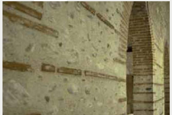
Historic internal wall repaired with Natural Hydraulic Lime mortar
