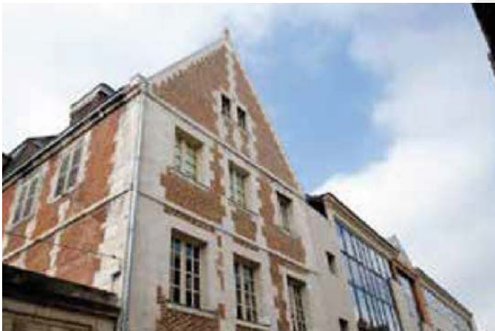
Natural Hydraulic Lime used for pointing new build construction
