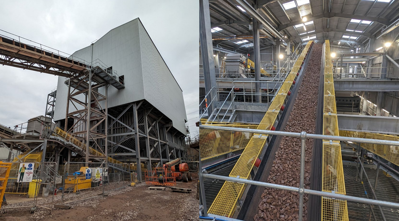
Mountsorrel Quarry's new permanent screenhouse
