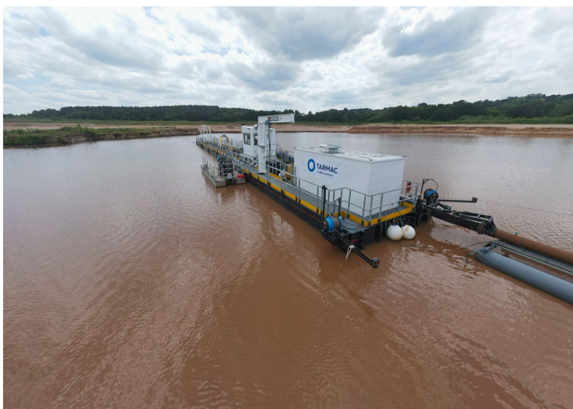
Example of a dredging operation (Crown Farm)
