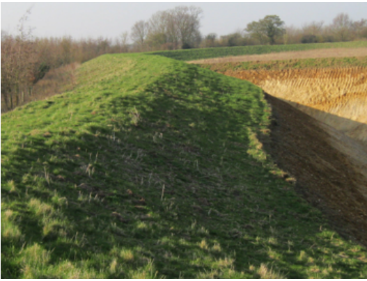
Example of a soil bund
