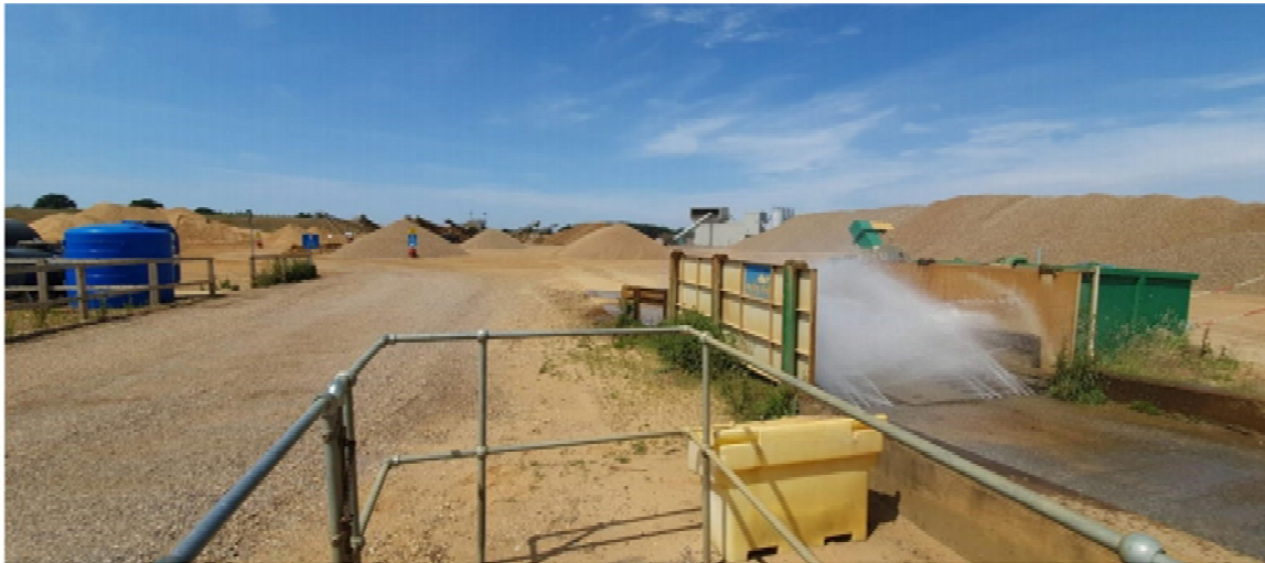
Wheel wash in use at Stanninghall Quarry
