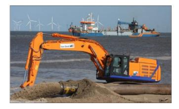
By using local offshore sources of sand and gravel for coastal defence work, large tonnages can be delivered rapidly by ship to replenish eroded stretches of coastline with minimal disturbance to local communities, providing environmental benefits, such as reducing trucks on local roads and protecting coastal communities.
