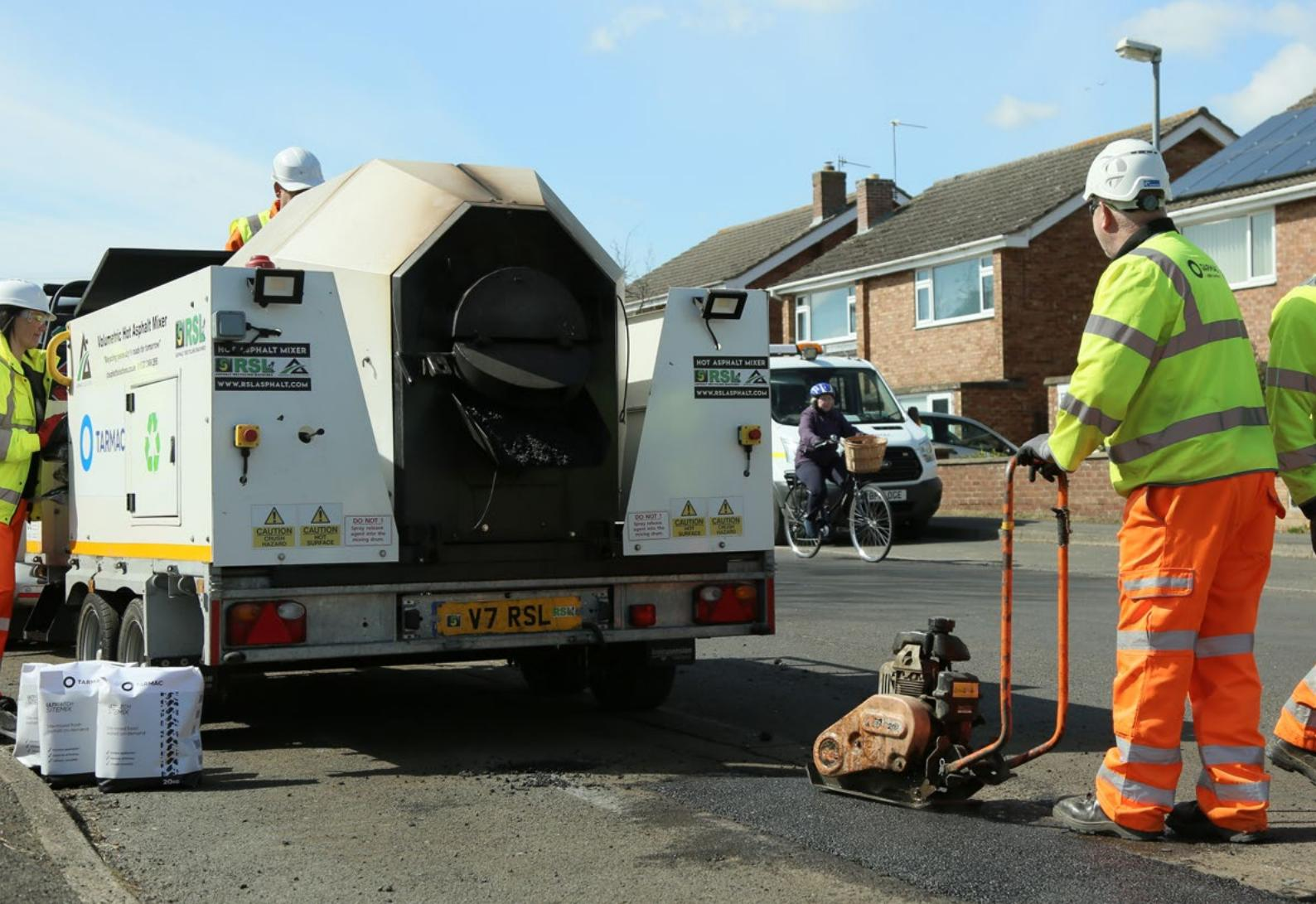
It was mixed on-site using a trailer-mounted asphalt heater and used at two different locations on neighbouring roads.
