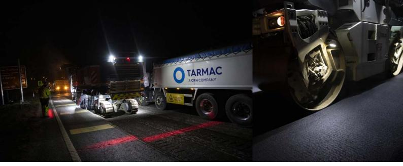
to reduce carbon emissions. This included using a warm mix asphalt binder and surface course in place of conventional hot mix asphalt and increased reclaimed asphalt planings (RAP) content. This helped to offset any additional carbon emissions from the SAMI layer and still deliver a 14% reduction in CO<sub>2</sub> emissions on materials.
